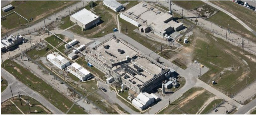
An aerial view of the 235-F Facility at the Savannah River Site. EM is set to decommission the building.
